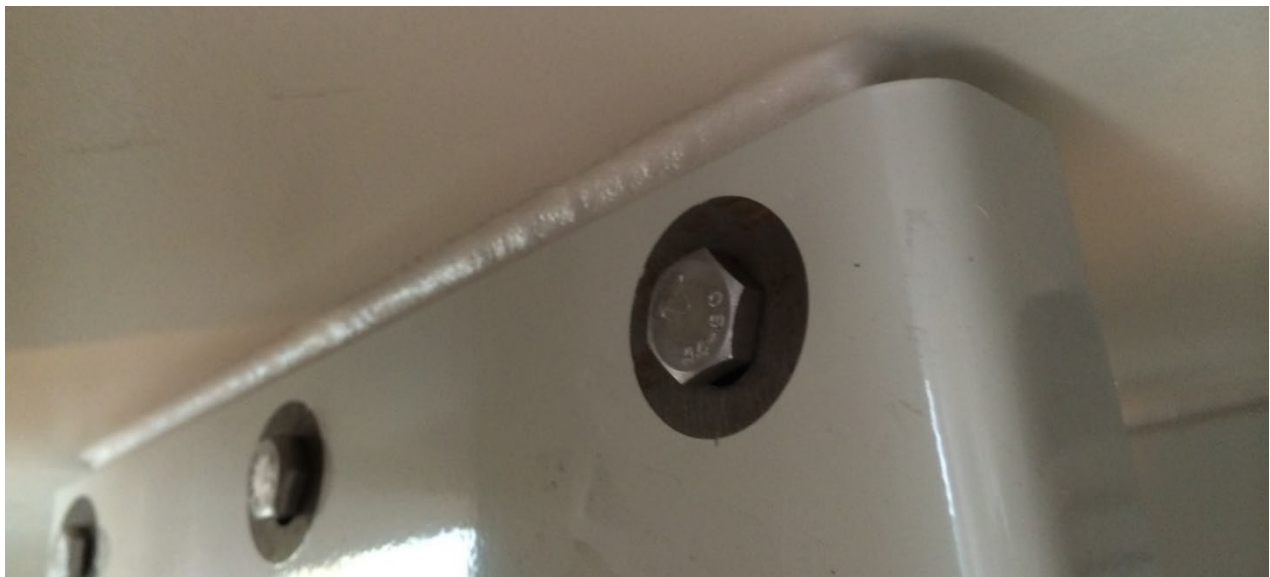
Fig. 2 The bolts on the flow separator plates.
